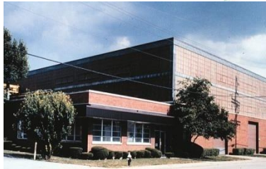
Steel Fabrication, Indiana, USA
