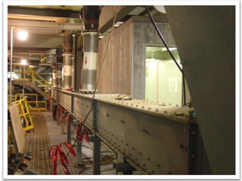
Continuous removal of Economizer Ash (Hawthorne Power Station)
