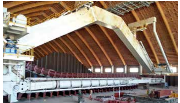
Erection of the portal by chain
