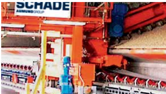
Discharge via impact idler table
