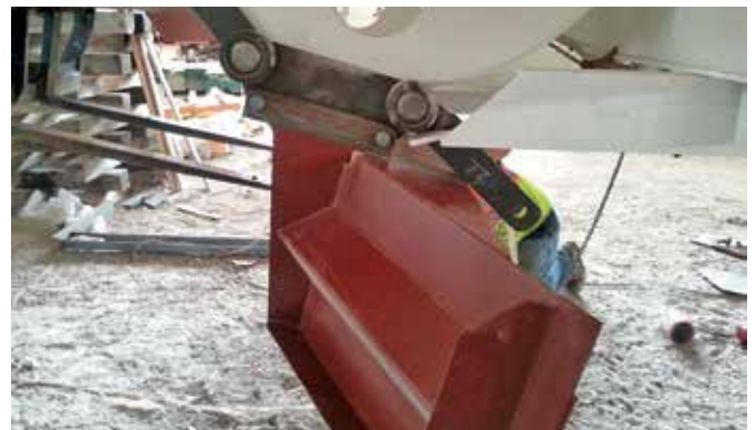
Installation of a shovel
