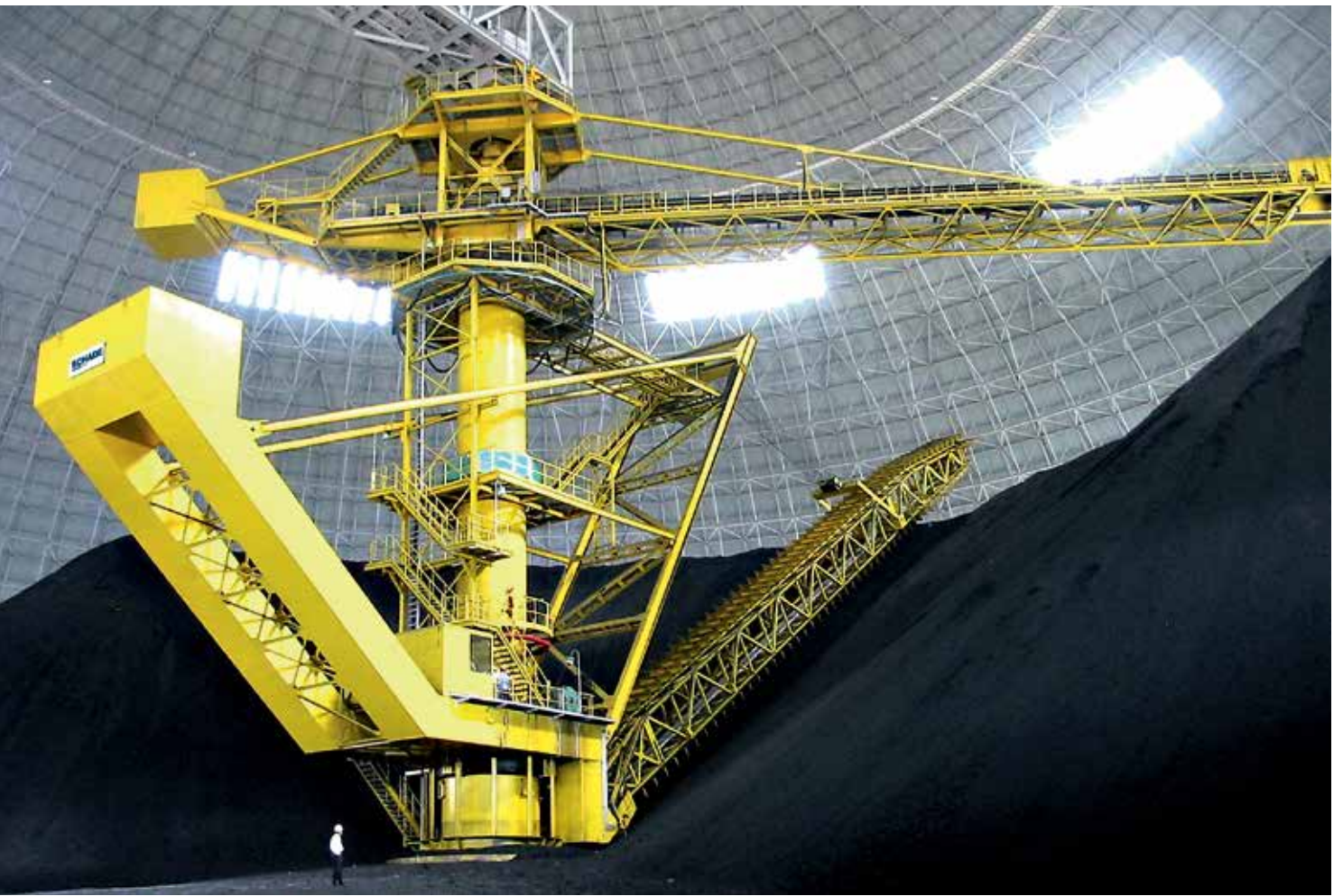
Circular Stacker Cantilever Scraper Reclaimer, dia 120 m, stacking 4,000, reclaiming 2,000 t/h, Coal
